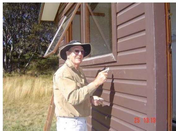
Len Hibble repairing weatherboards around window frame.
