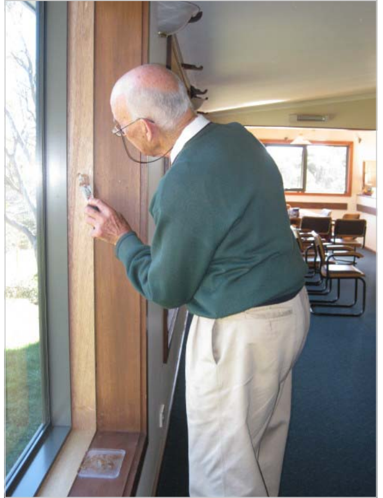
Ed Pietor filling one of the 600 nail holes left by the installers
