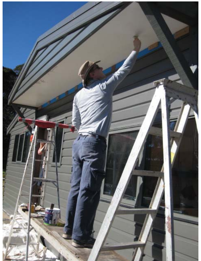
Ed Pietor filling one of the 600 nail holes left by the installers
